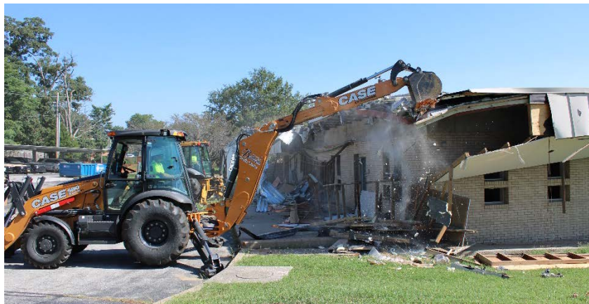
Demolition of the old police building in Vlasik Park. This area will be returned to the park as green space as part of the Public Works Yard Reconfiguration project.
