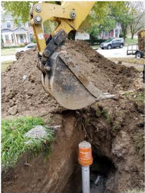
Sewer Lateral Repair: City of Manchester allows for settling after the repair, making a second visit to regrade. This avoids unwanted sunken areas in the yard.
