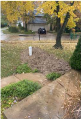
Sewer Lateral Repair: City of Manchester allows for settling after the repair, making a second visit to regrade. This avoids unwanted sunken areas in the yard.
